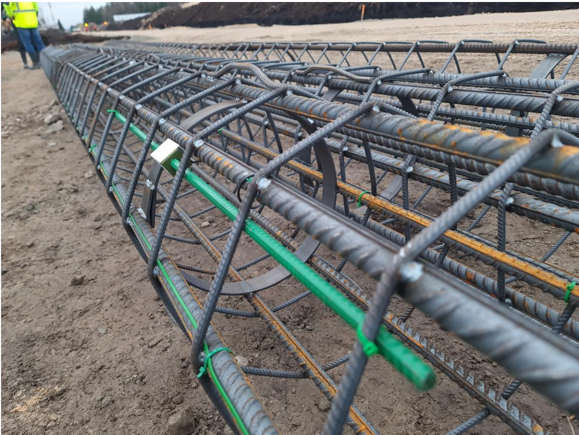
Picture 1 SlabControl 5.0 installed on wind park construction site for future loadbearing monitoring and pile performance
